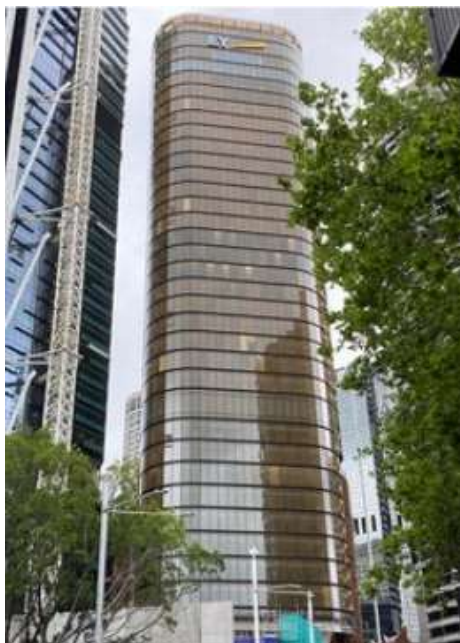
Figure 4. Wooden blinds made from acetylated wood in a high-rise building in Sydney, Australia (Evans et al., 2022)
