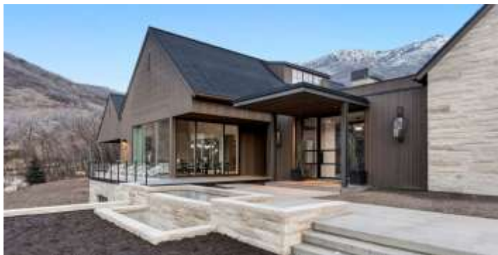
Figure 3. Construction from thermally treated wood (URL-2,2024)
